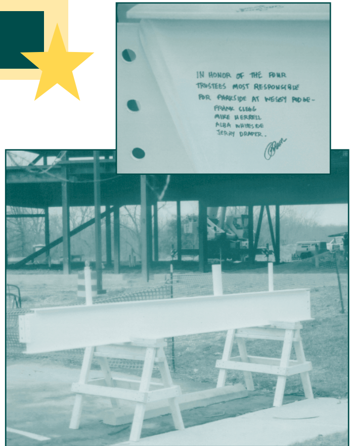
Photos taken of the “Topping off” Dedication that was held in the winter of 2005. In honor of their work, the names Frank Clegg, Jerry Draper, Mike Herrel and Alba Whiteside were written on the last and top beam that was raised at the “topping-off” ceremony.
